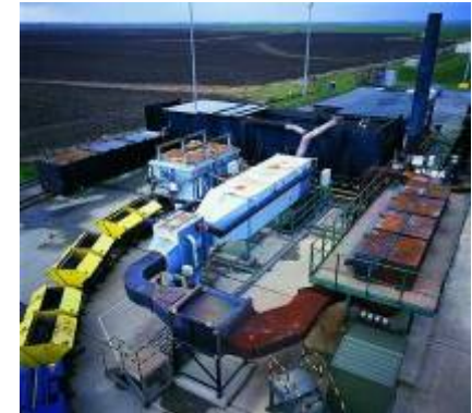
Avocet Explosive Waste Incineration site (2 x rotary furnaces) .
